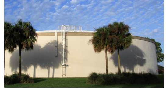
Water Storage Tank at Water Treatment Plant 3
