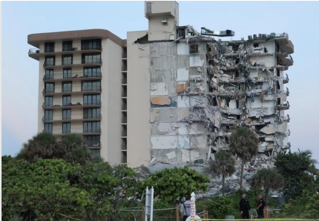
Champlain Towers South in Surfside, Florida
