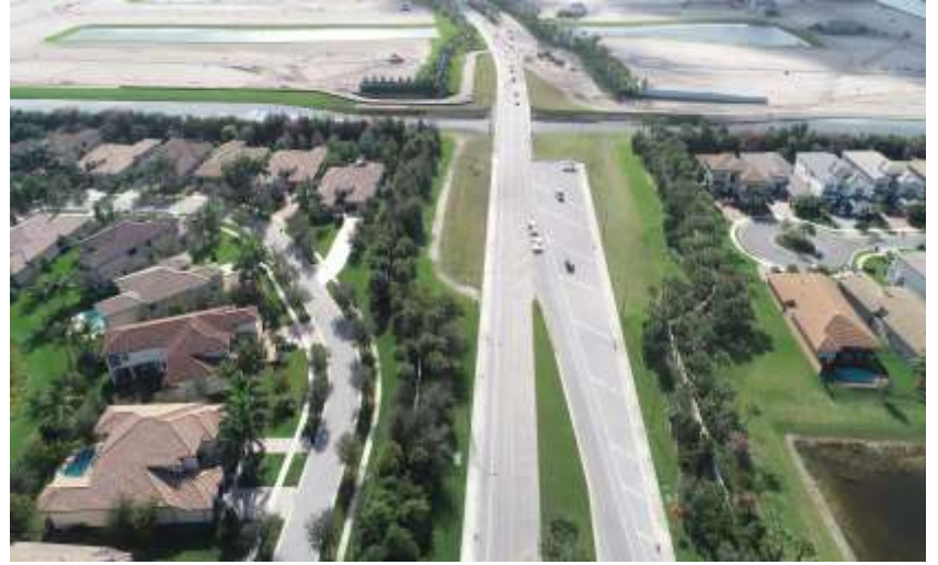
L-38 CANAL BRIDGE
