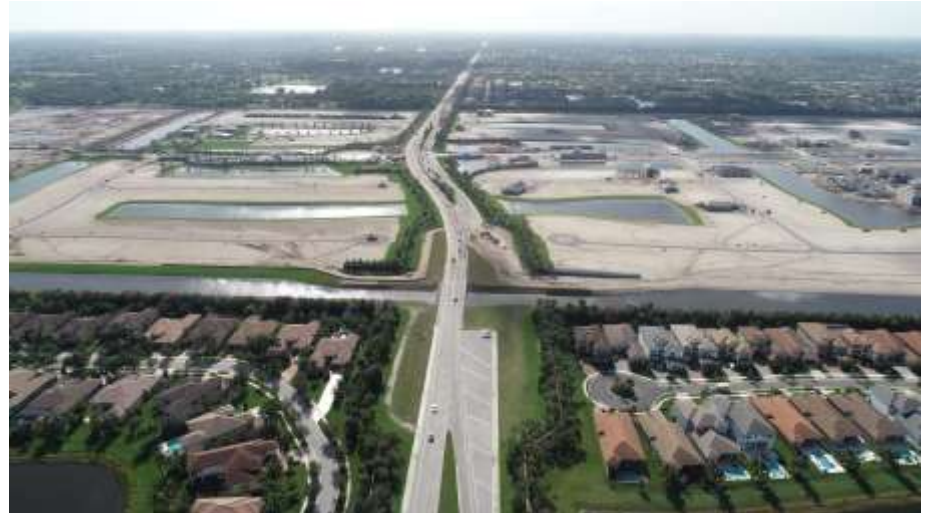
THE BRIDGE AT L-38 CANAL
